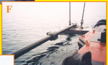
F: detail of the sinker (40 tonnes in air) linked to the metallic structure
