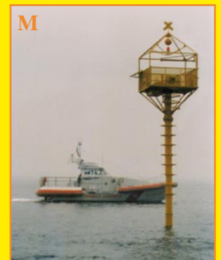
M: the finished platform is inspected for the first time by the Italian Coastguard!
