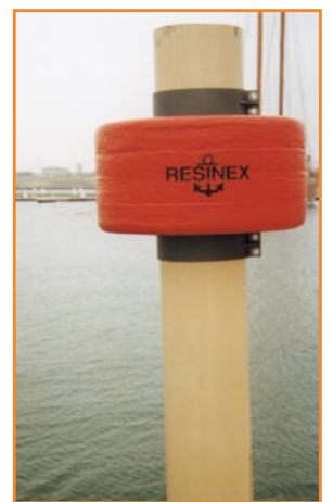
Pipe fender installed
