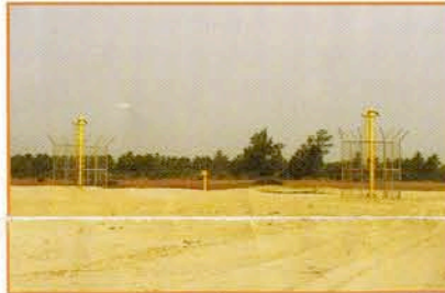
Onshore signals protected from intrusion
