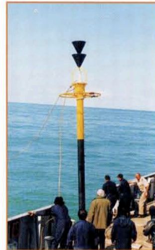
Positioning of south cardinal elastic beacon
