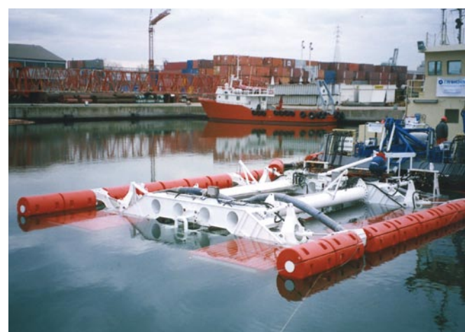
The complex shallow water trenching machine.
