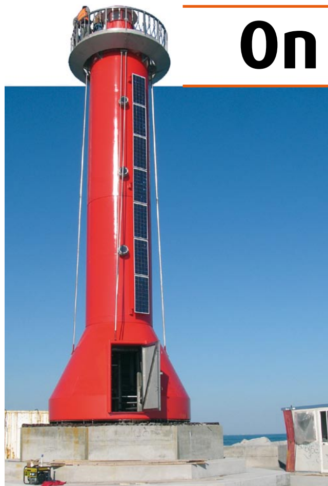
The light tower at the extreme east of Malamocco dam. Below right, the tall stainless steel land beacon positioned on the opposite side.
