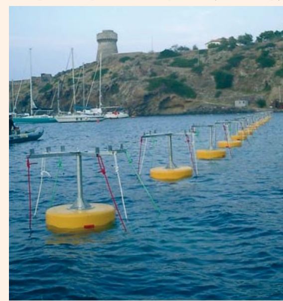
Capraia: Resinex buoys with a special "rope keeper" system (Bollani project).
