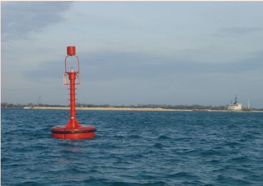
Light buoys in the Malamocco canal.
