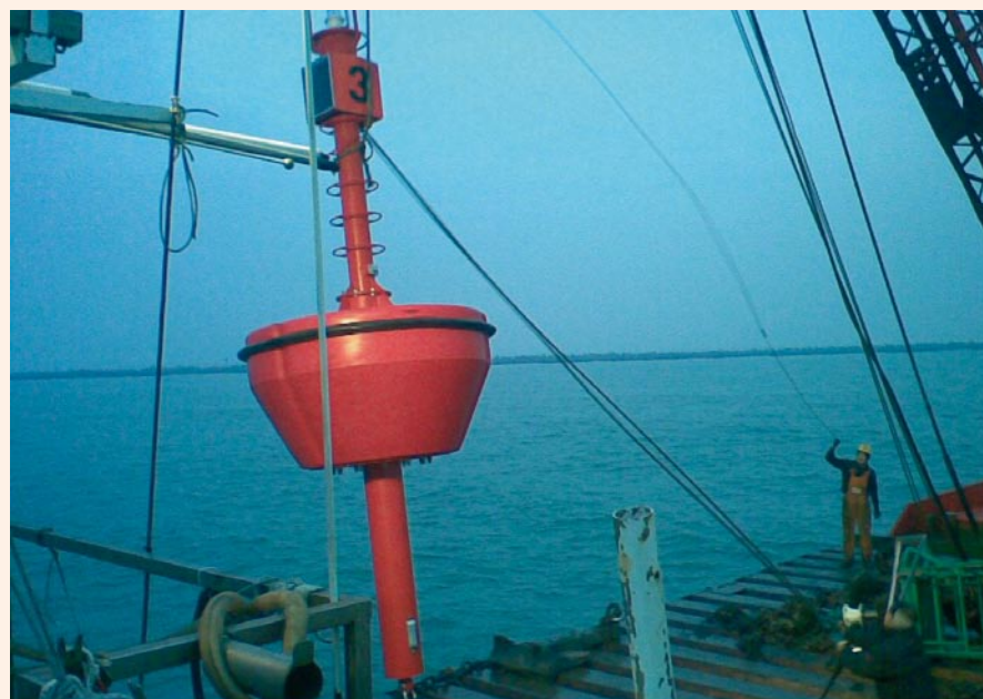
Installation of large light buoys in the Ravenna outer port.
