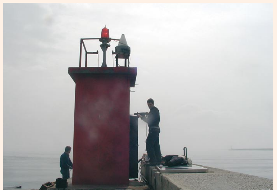
Port of Triest: maintenance of lantern and Racon at the lighthouse.
