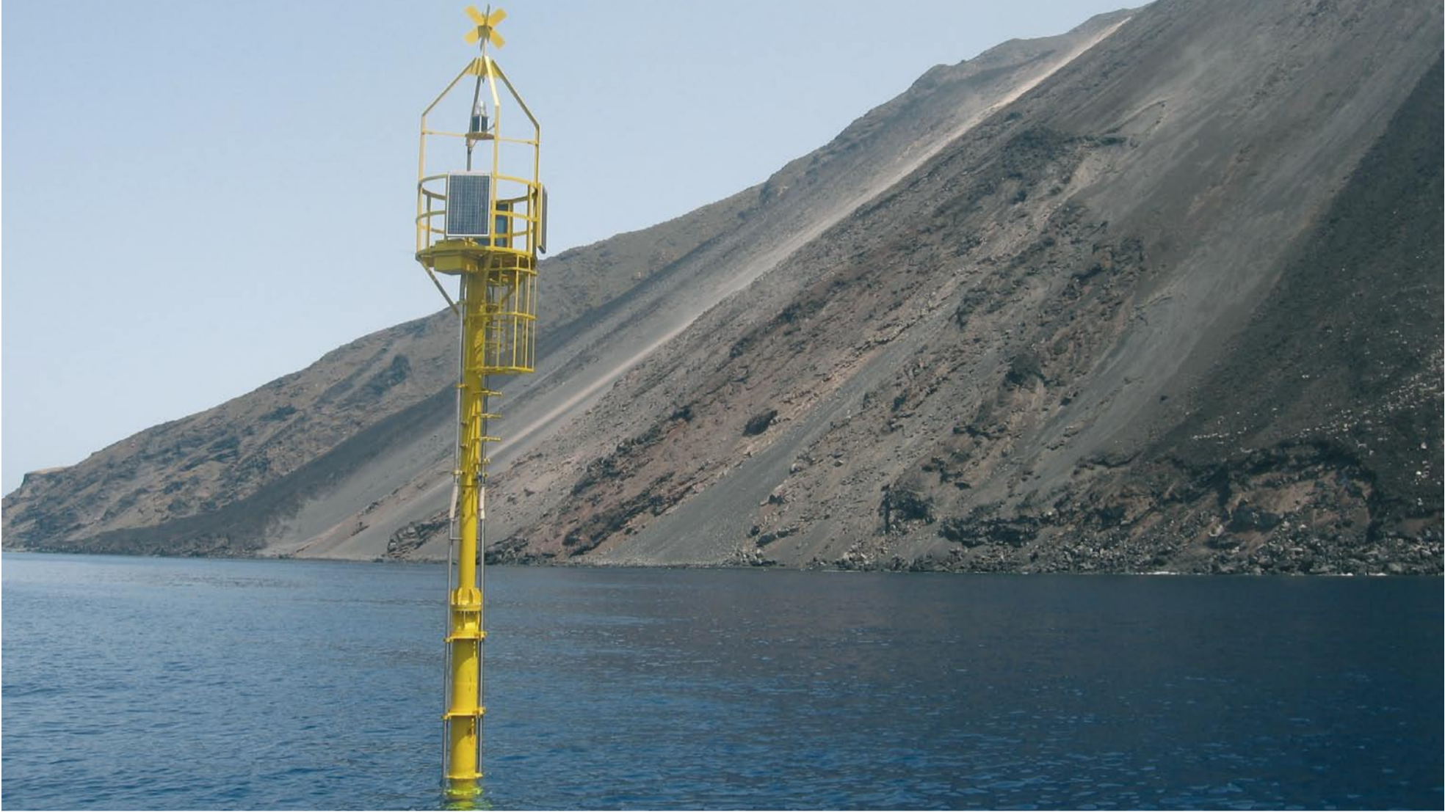
The beacon is equipped with many monitoring systems powered by solar panels.
