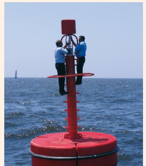
Twelve Resinex light buoys with 3 meter diameter float were recently located in the Alexandria port (Egypt) as a replacement of old buoys.
