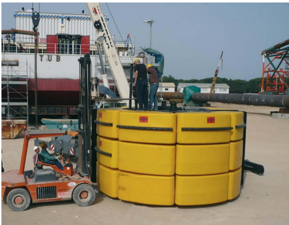
Final assembly onshore, final details on board and the load test of the Ravenna's giant.
