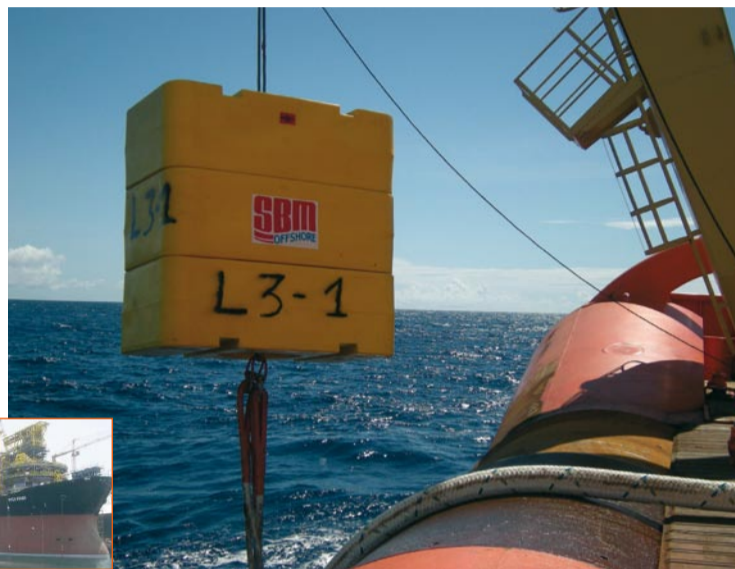
Up: Resinex synt buoys NB 2.1 tons in operation underwater. Left: the installation of the SBM support buoys in the Frade field (Brazil).
