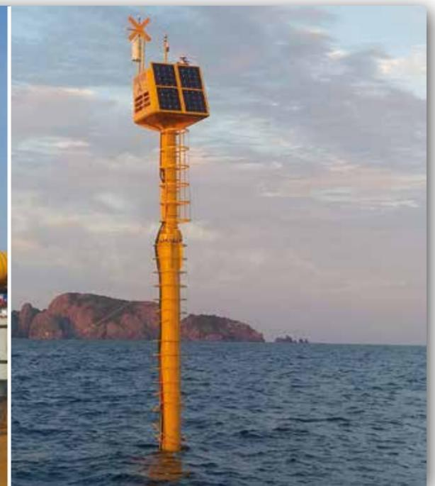
Then, ad hoc elastic beacons have been projected with a float of 4.3 m of diameter, 2.5 m of height and 16 tonnes of net buoyancy. Beacons have an average height of 51 m, a focal plane of 14 m to keep the visibility against high tide variations and have been realized for depths of 34.5 m, 34.6 m and 35.5 m.
