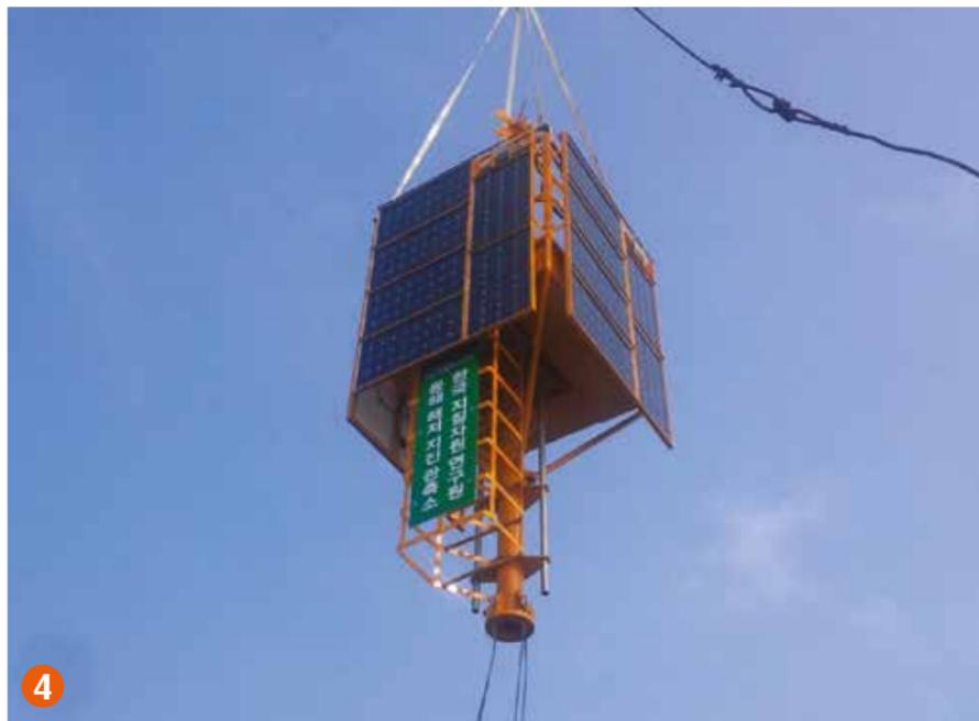
The beacons are equipped with a huge turret (2x2 metres), able to host the power system (solar panels and batteries) and the electronic equipment which controls the devices placed on the sea bed by Guralp Systems Ltd, for surveying the geophysical activity and the transmission of data to-land.
