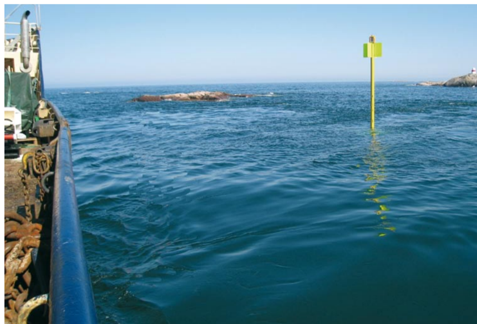
Above: the Resinex special elastic beacon during the assemble in Västervik port. Below: the installed elastic beacon near the rock outbreaks.
