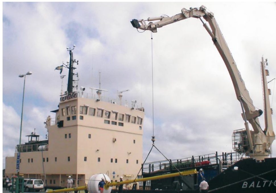
Above: the Resinex special elastic beacon during the assemble in Västervik port. Below: the installed elastic beacon near the rock outbreaks.
