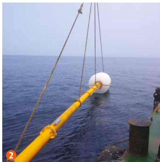
Photo 1, 2 and 3: assembly of the lower part at sea. The beacon structure is more than 40 metres long.
