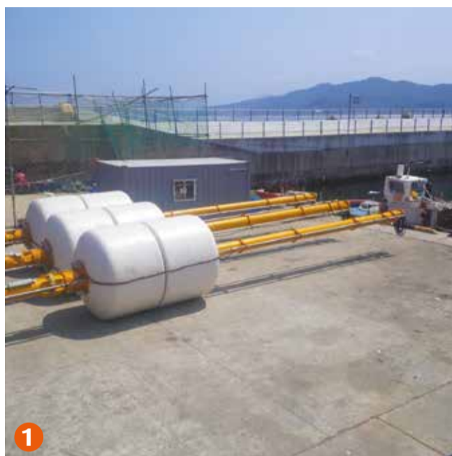
Photo 1, 2 and 3: assembly of the lower part at sea. The beacon structure is more than 40 metres long.
