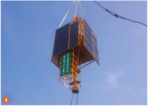
The beacons are equipped with a huge turret (2x2 metres), able to host the power system (solar panels and batteries) and the electronic equipment which controls the devices placed on the sea bed by Guralp Systems Ltd, for surveying the geophysical activity and the transmission of data to-land.
