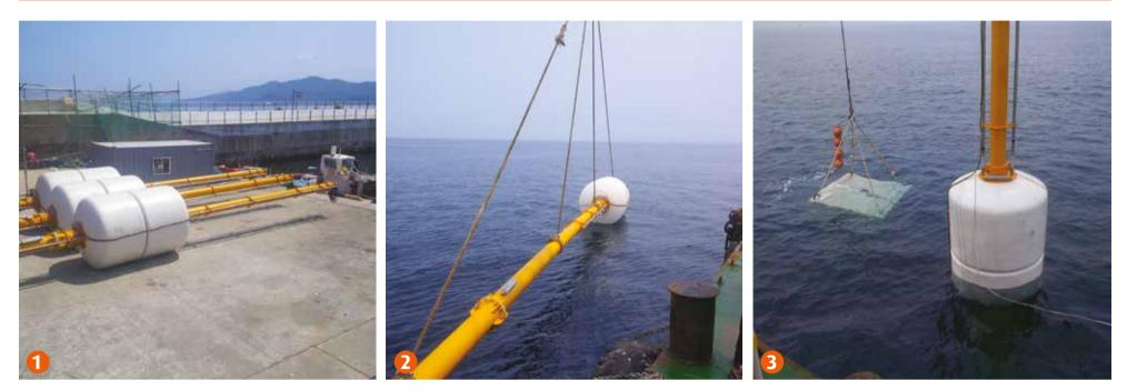
*Photo* **1**, **2** *and* **3***: assembly of the lower part at sea. The beacon structure is more than* 40 *metres long.*
