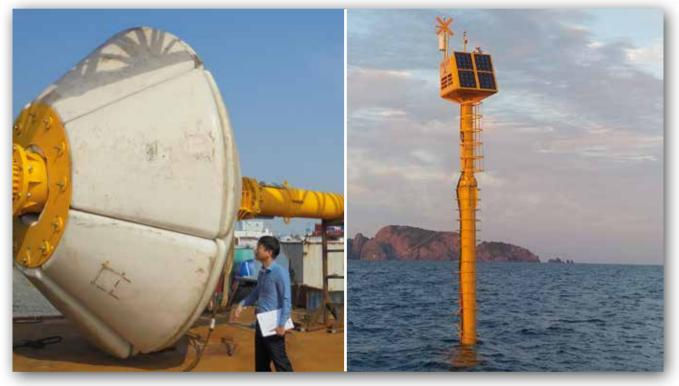
Then, ad hoc elastic beacons have been projected with a float of 4.3 m of diameter, 2.5 m of height and 16 tonnes of net buoyancy. Beacons have an average height of 51 m, a focal plane of 14 m to keep the visibility against high tide variations and have been realized for depths of 34.5 m, 34.6 m and 35.5 m. They are also complete of an upper platform on which the necessary instruments for the monitoring are applied.
