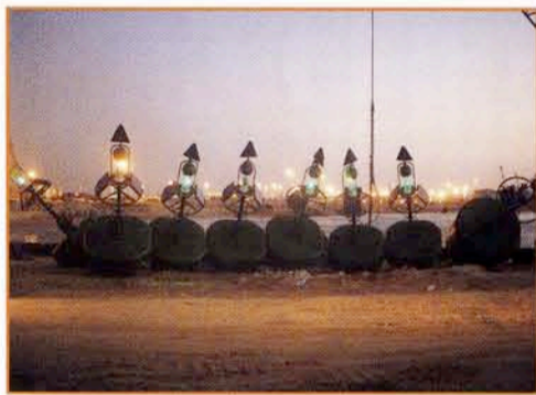
Light test of the buoys before installation
