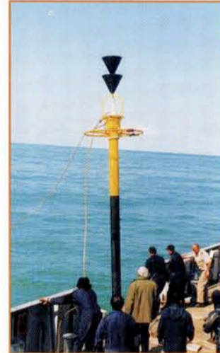
Positioning of south cardinal elastic beacon
