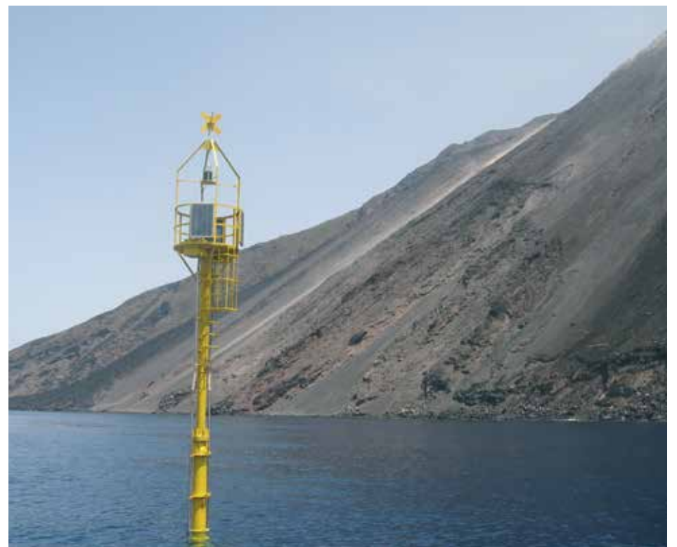
The beacon is equipped with many monitoring systems powered by solar panels.
