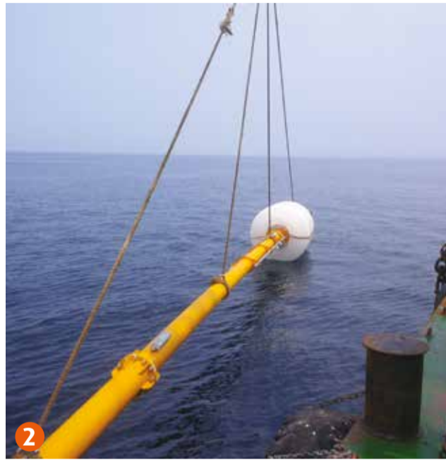
Photo 1, 2 and 3: assembly of the lower part at sea. The beacon structure is more than 40 metres long.
