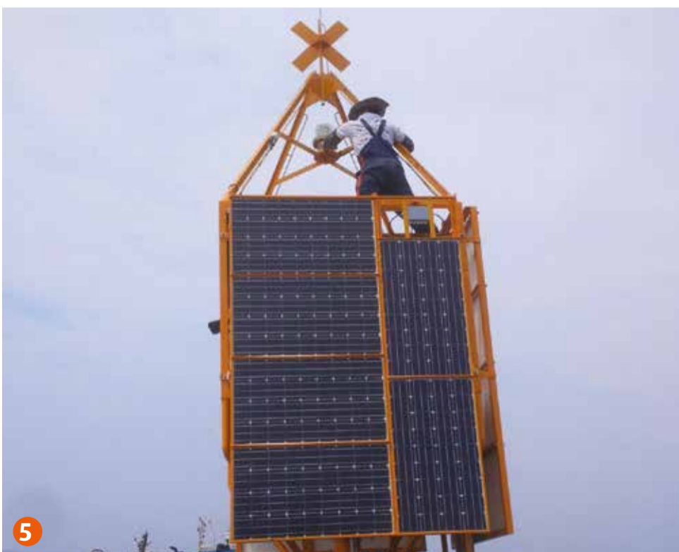
Photo 4, 5 and 6: assembly of the upper part, able to host the power system and the electronic equipment.
